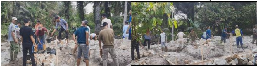
Figure 2. Residents work together to build the foundation of a house
