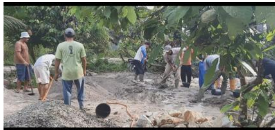
Figure 1. for making cement mixture for foundation
