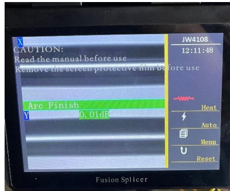
Figure 3. Fiber Optic Cable Fusion Splicer Splicing Result
