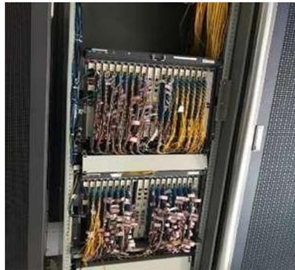
Figure 3. Optical Line Terminal
